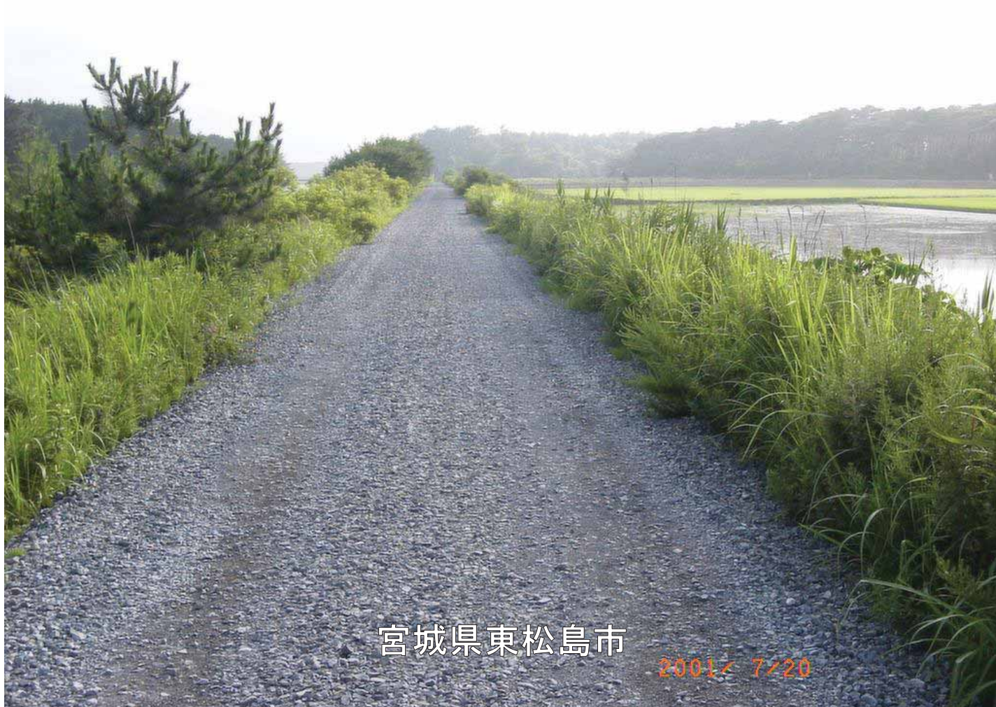
3003_1_011_003956_高橋親夫_2001.7.20_北上運河(野蒜築港跡～浜須賀)
